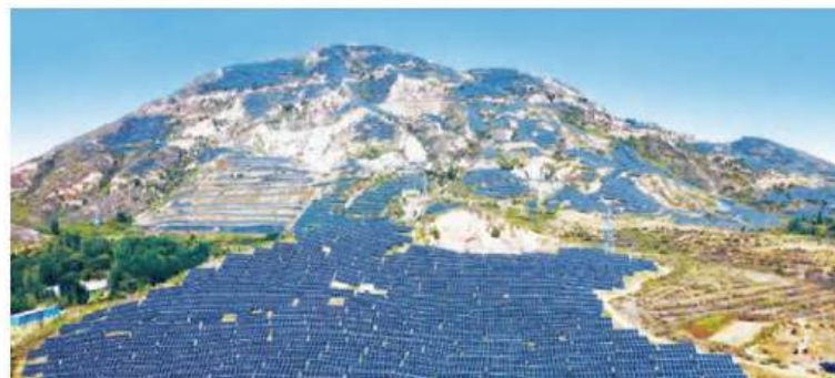
Location: Croatia Capacity:120kW/200kWh
