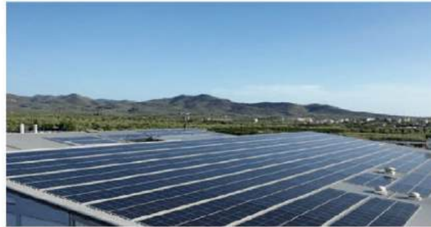
Location: South Africa Capacity: 60kw /100kWh
