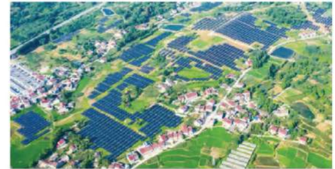
Location: Suriname Capacity:250kW/1MWh
