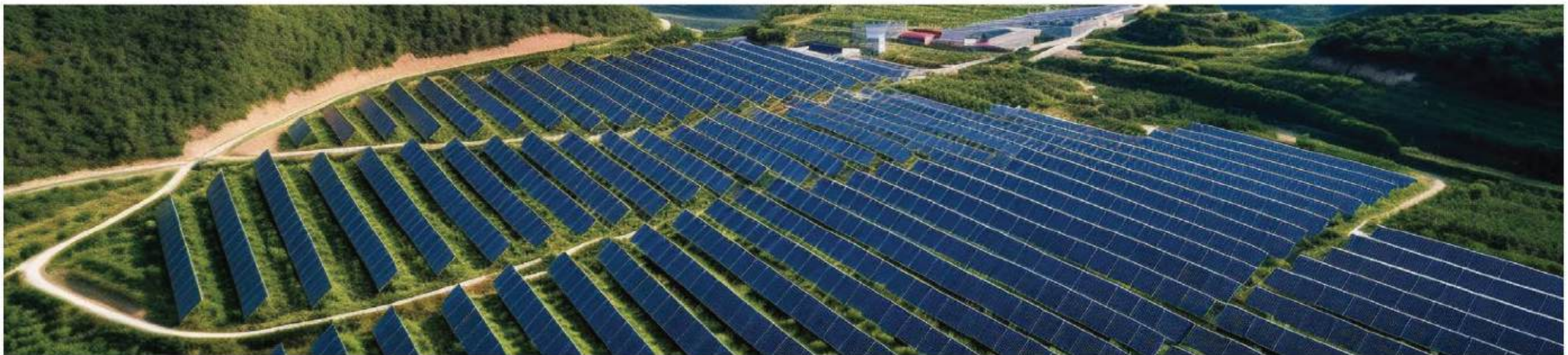
Location: South Africa Capacity:750kW/1.5MWh
