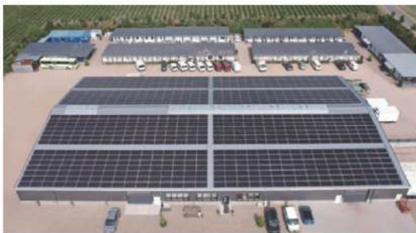
Location: South Africa Capacity:1MW/1.3MWh
